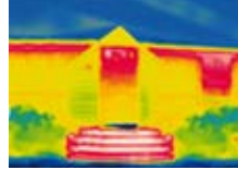
Building: Heat Loss
